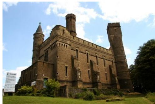
Figure 65: The Castle Climbing Centre, Manor House
